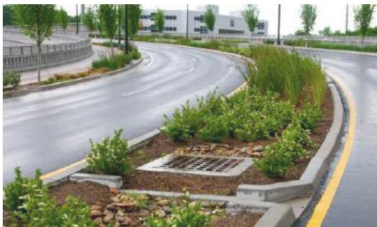
Boulevard streetscape, sidewalk amenities, and stormwater improvements
