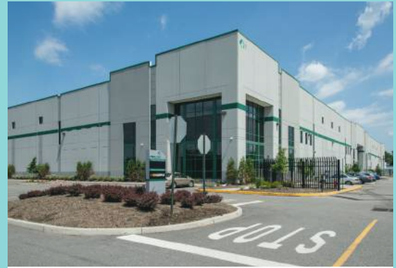
Light industrial warehouse
