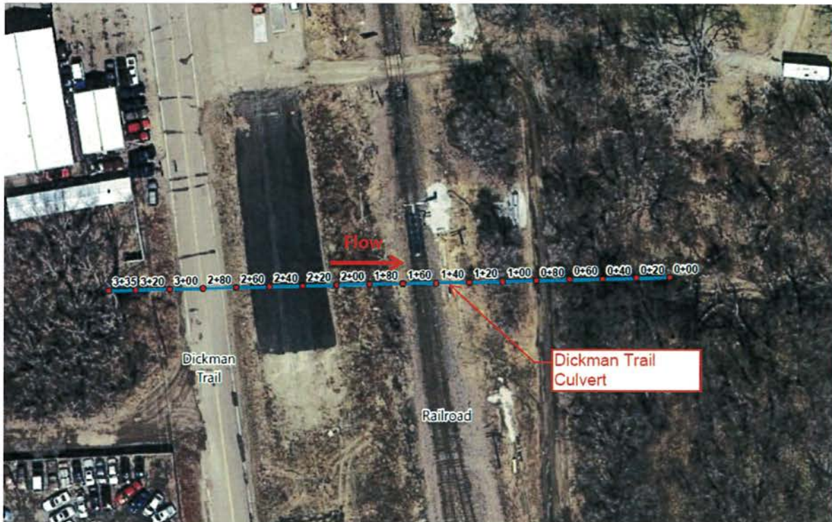
Figure 1-1 Dickman Trail Culvert
