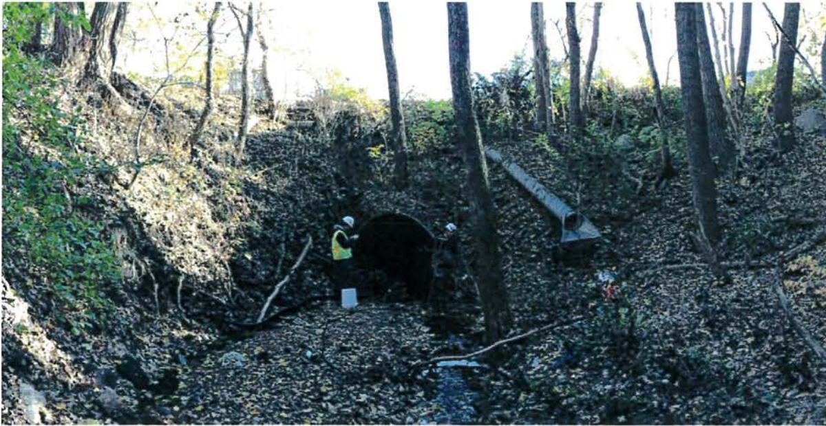
Figure 4-2 Existing Vegetation at the Culvert Inlet
