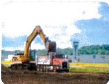
Holman Field St. Paul Downtown Airport - RW 14-32/RW13/31 Reconstruction
