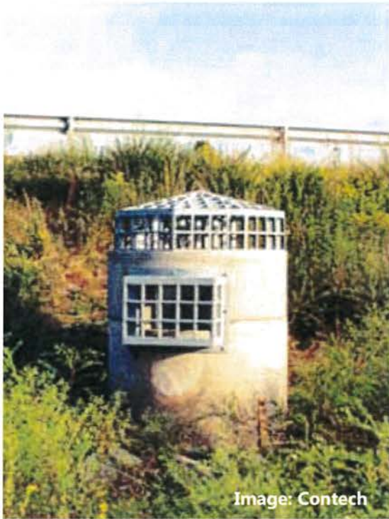
Figure 5-2 Concrete Inlet Structure
