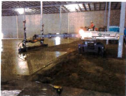
Fulford Warehouse – Lakeville, MN
