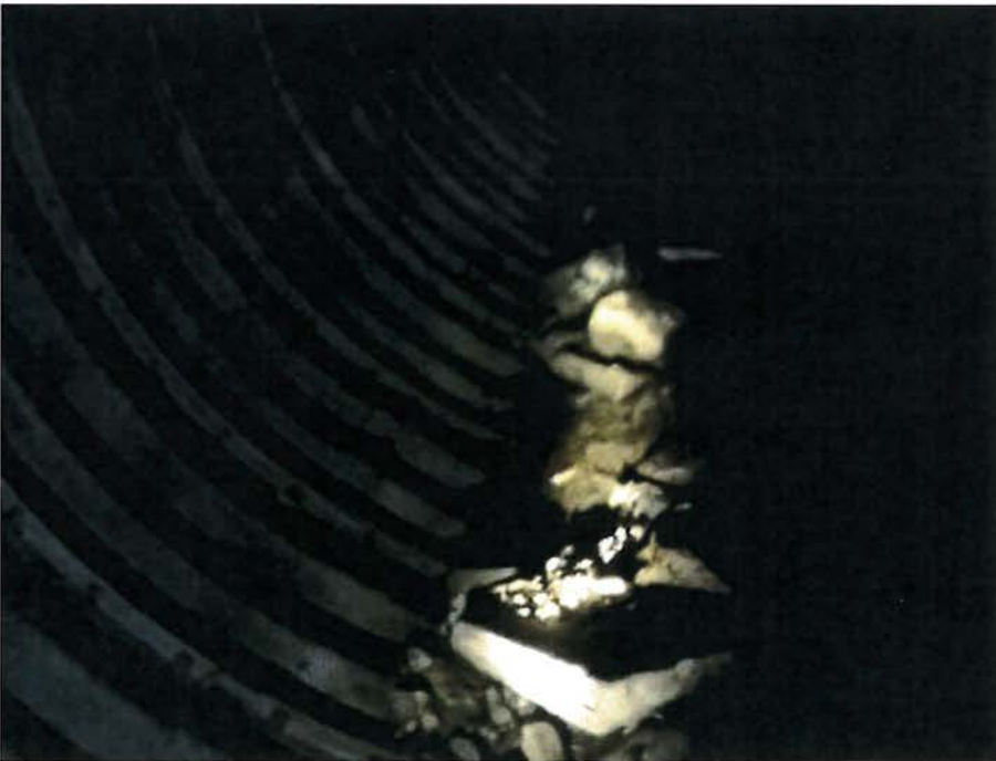
Figure 4-7 Settled Gravel and Deposits
