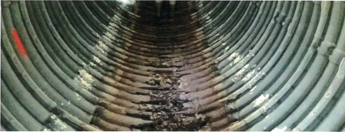
Figure 4-6 Typical Corrosion
