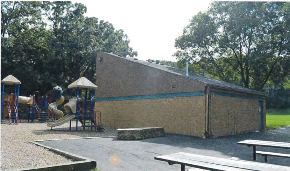
Existing Warming House Year constructed: 1980 To be removed. New picnic shelter to have storage and restrooms.
