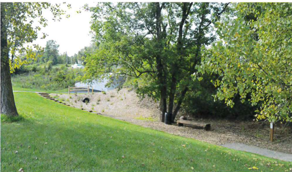
Existing Tunnel, Raingarden, and Disc Golf Hole Year constructed: 2010 Area to continue as stormwa- ter drainage with raingarden. Tunnel to remain as-is. Disc golf holes to be re-organized for full course to be contained within North Valley Park.
