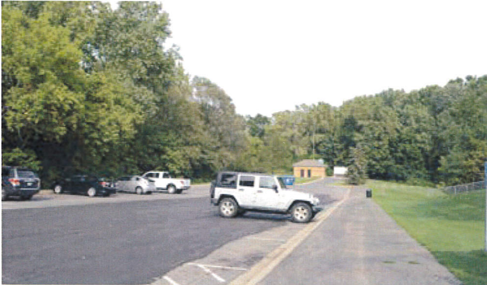
Existing Parking Lot Year constructed: To remain with new striping, extension to add 22 spaces.
