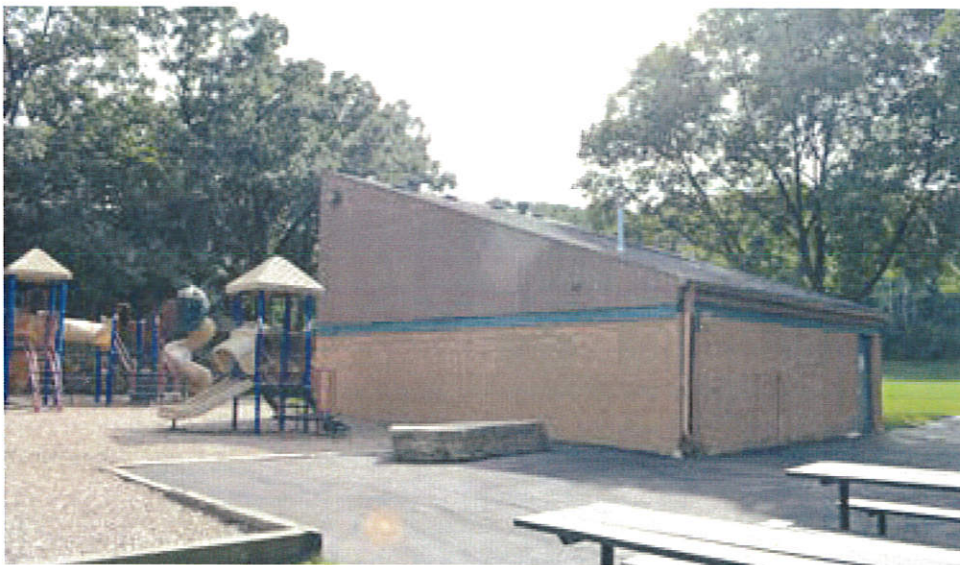
Existing Warming House Year constructed: To be removed. New picnic shelter to have storage and restrooms.
