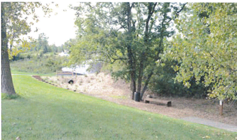
Existing Tunnel, Raingarden, and Disc Golf Hole Year constructed: Area to continue as stormwa- ter drainage with raingarden. Tunnel to remain as-is. Disc golf holes to be re-organized for full course to be contained within North Valley Park.
