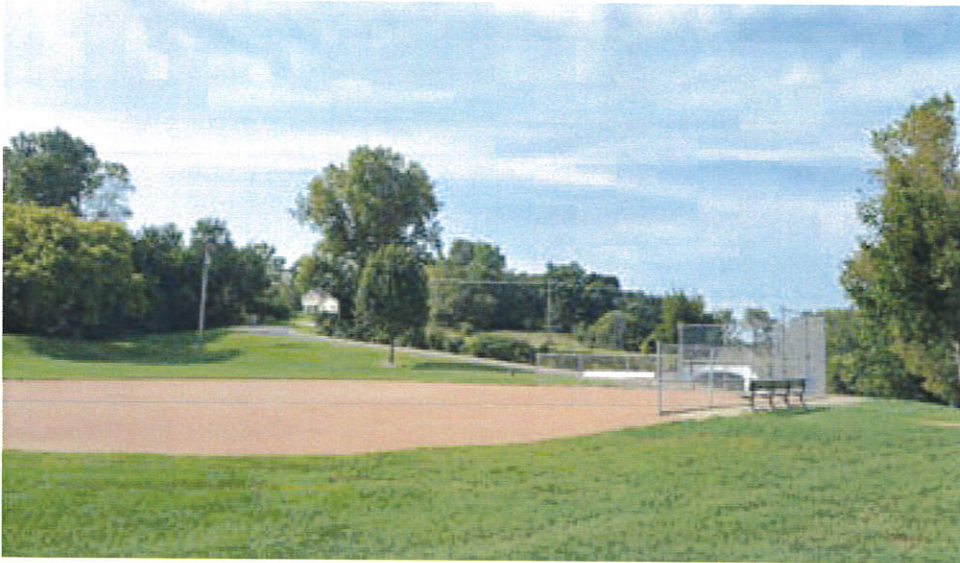
Existing Ballfield Year constructed: Fencing, aglime, bench to be removed. Area to be converted to pollinator lawn and regraded for the picnic shelter and performance area.
