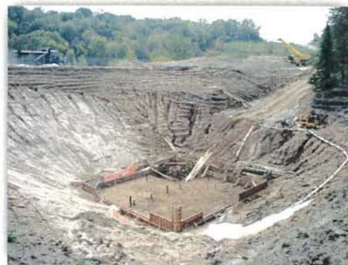
2008 Argenta Hills Lift Station Construction
