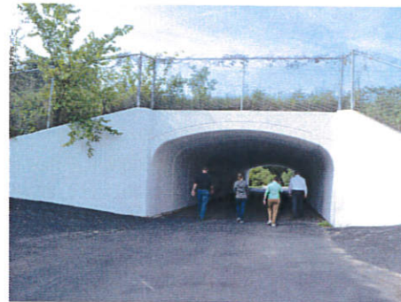
The pedestrian tunnel under 70th Street between North and South Valley Parks after a fresh coat of paint
