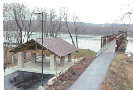
Swing Bridge Park
