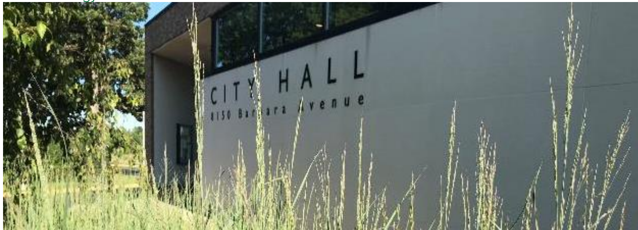
Figure 17: Inver Grove Heights' City Hall. This building uses a ground-source heat pump (geothermal) to meet energy needs.
