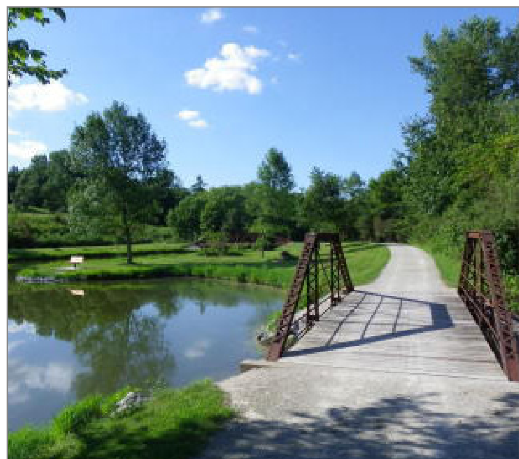
Stormwater treatment as an amenity
