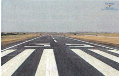
Figure 39: Completed construction of the overlay for Runway 17/35 at Meacham International Airport.
