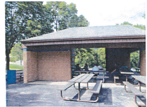
Existing picnic shelter
