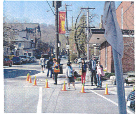
Tactical approaches to new facilities can be low-cost and temporary. The example above demonstrates how a temporary crosswalk bump out is being tested for future improvements
