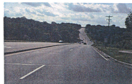
Existing conditions at the intersections of 70th Street and Cahill Ave (Top), and 70th Street at North and South Valley Parks
