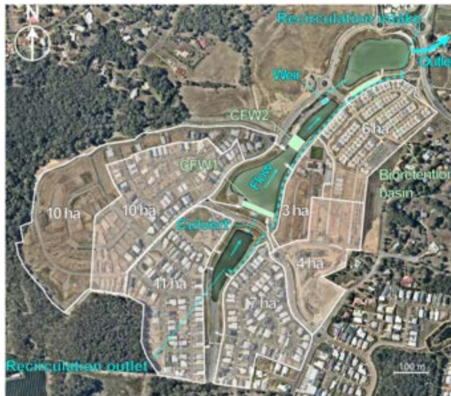
Fig. 1. Aerial view of the “Parklakes 2” development, with two constructed floating wetlands, CFW1 and CFW2, installed in a 2.6 ha lake treating stormwater runoff from a 45-ha urban development area (Nearmap, 17. Feb. 2017).
