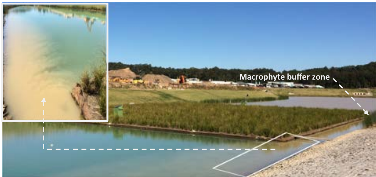
Fig. 5. Visual observation of untreated stormwater runoff short circuiting at the edge of the second constructed floating wetland, CFW2.
