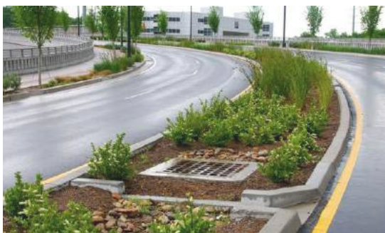
Boulevard streetscape, sidewalk amenities, and stormwater improvements
