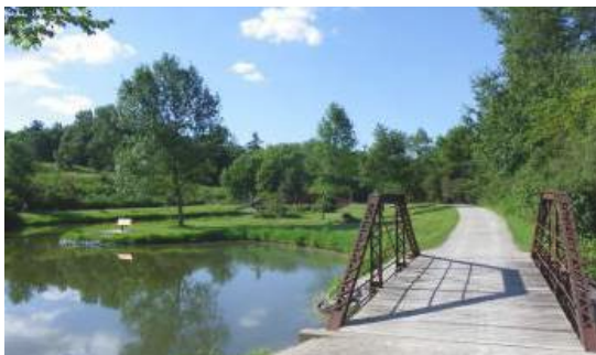
Stormwater treatment as an amenity
