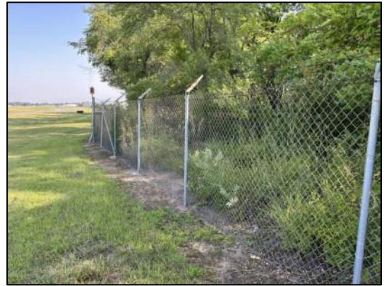
Photo 1 – Existing Airport Perimeter Fence
