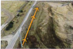
b Transmission Power Poles may be impacted by construction. These locations and impacts will be identified and impacts minimized through the Utility Coordination and SUE process
