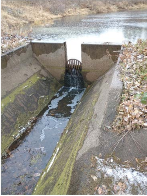
T-8 Pond outlet structure weir
