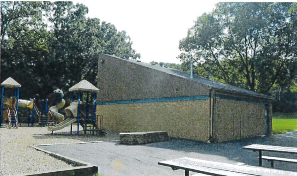
Existing Warming House Year constructed: 1980 To be removed. New picnic shelter to have storage and restrooms.
