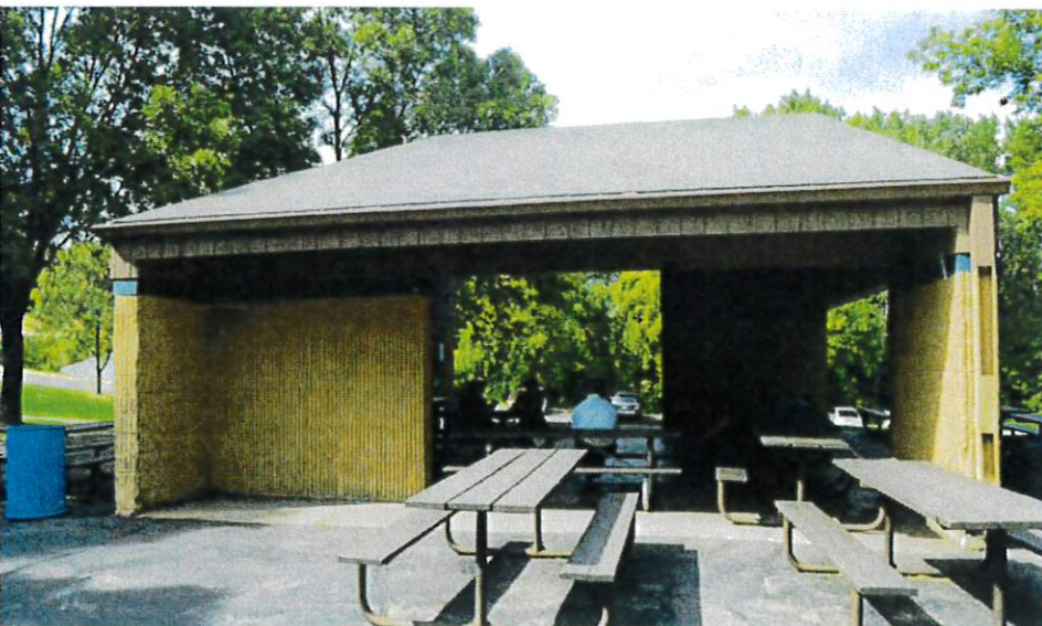
Existing Picnic Shelter Year constructed: 1980 To be removed and replaced in a new location.
