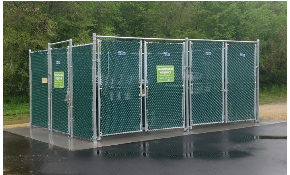
Dakota County Transportation Garage, Hastings
