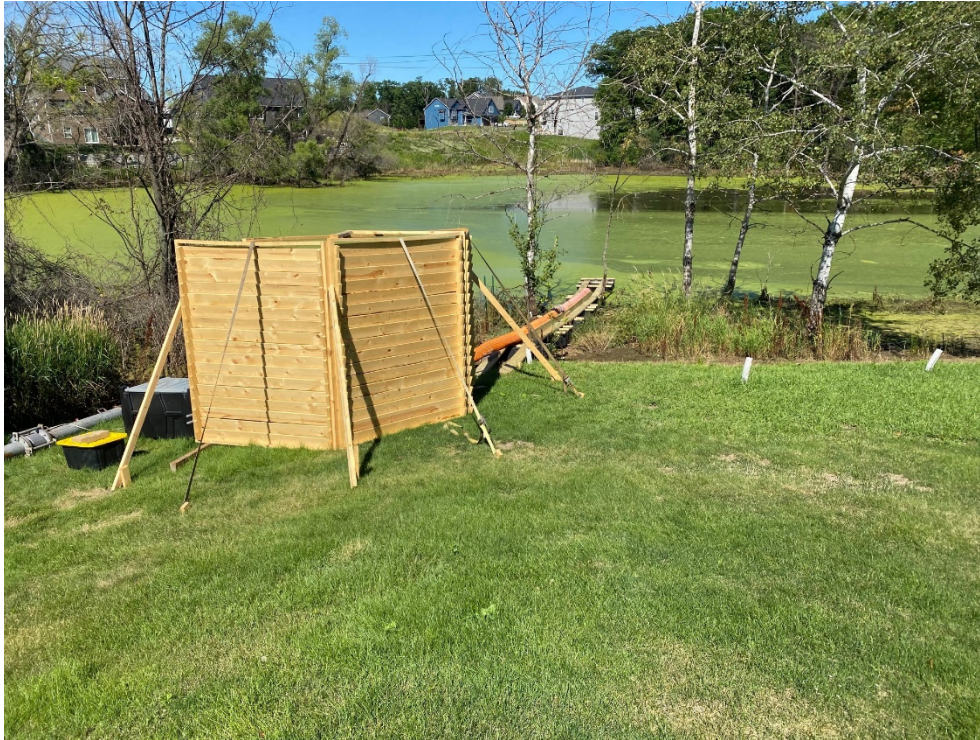
Figure 8 IGT-B-3 Basin after Completion of Temporary Pumping Project
