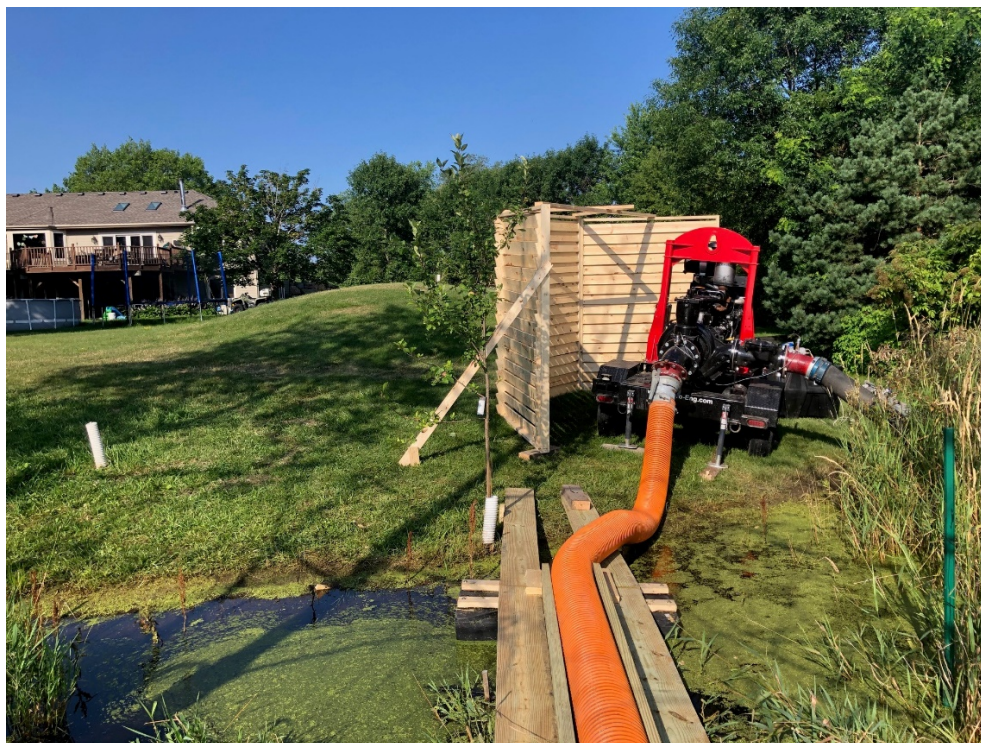
Figure 7 Portable Pump in Operation with Noise Shielding
