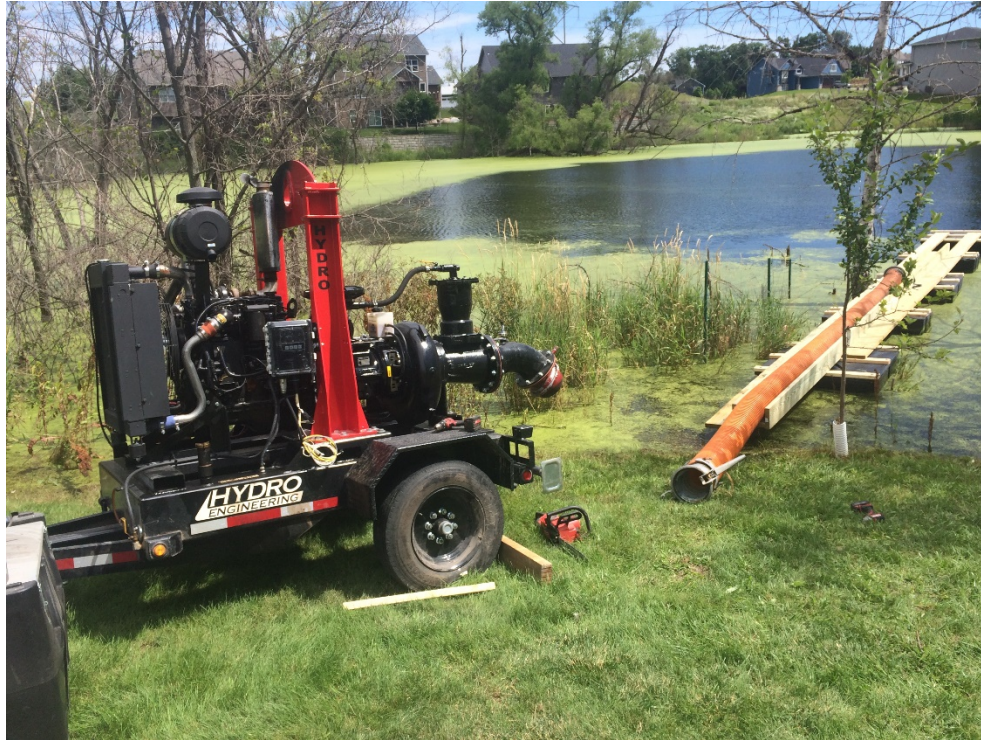
Figure 6 Portable Pump and Intake Pipe Setup, Before Starting Pumping
