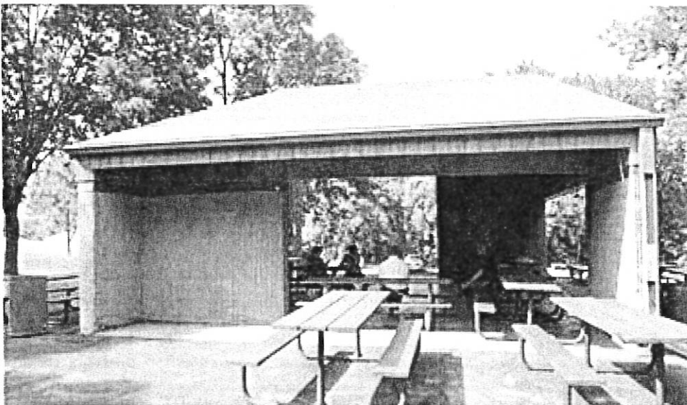
Existing Picnic Shelter Year constructed: To be removed and replaced in a new location.
