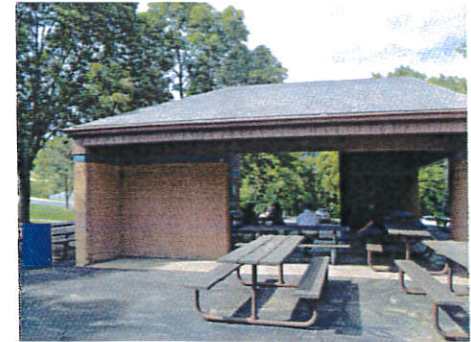
Existing picnic shelter
