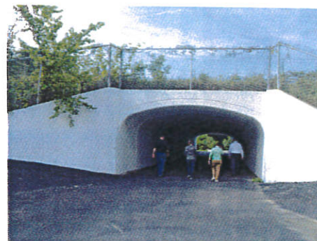
The pedestrian tunnel under 70th Street between North and South Valley Parks after a fresh coat of paint
