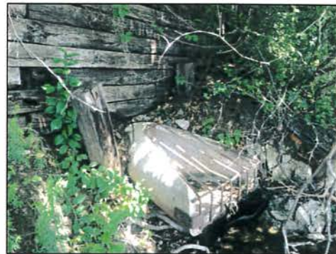
Flared End and Retaining Wall
