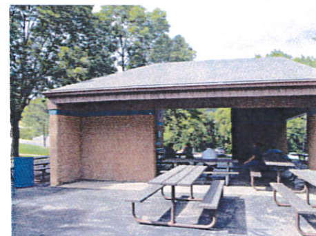
Existing picnic shelter
